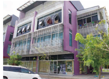
The office is located on the 1st floor of a new building. 新築ビル1階に入居するオフィス
